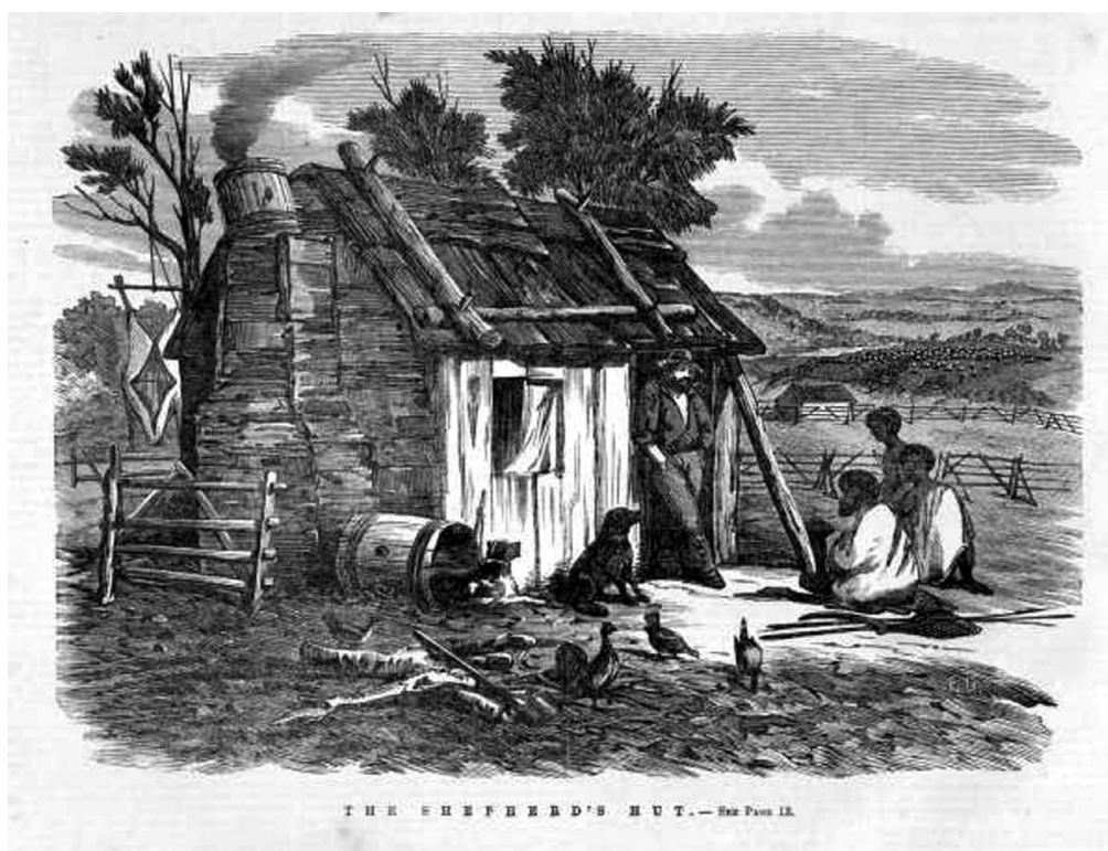
Figure 2. The shepherd's hut showing bark construction with roof weighted down by pegged logs. Leaning against the bark chimney is a mortised hurdle with characteristic diagonal braces. A yard made of hurdles supported by forks is on the right rear. Two details are unrealistic: chickens are unlikely as no contemporary observer recorded them; and relations with Aborigines were hostile more often than not so the presence of spears is problematic.
