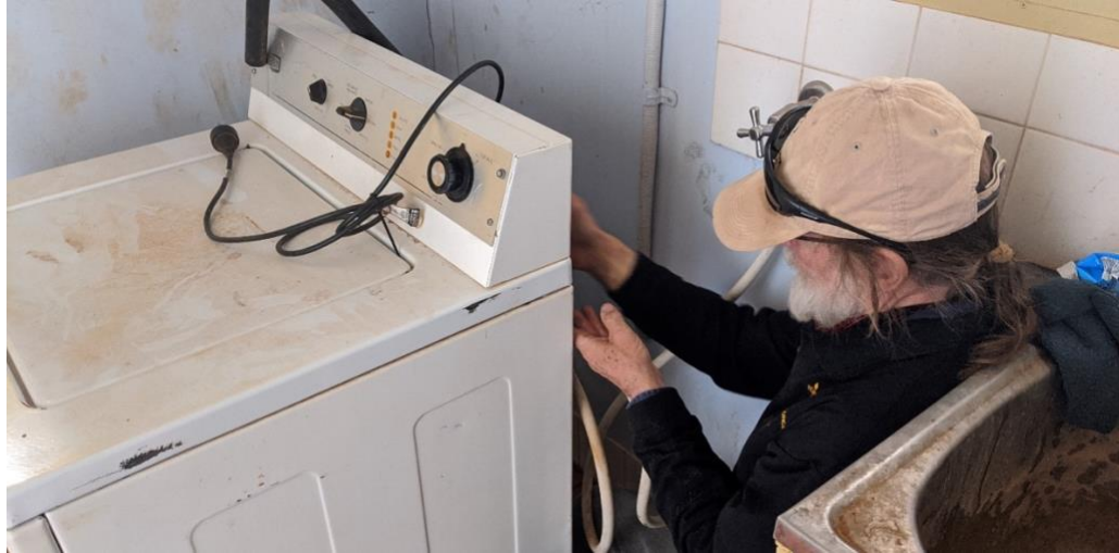
Figure 2: Scott Robinson installing a Maytag washing machine. Image: Liam Grealy
